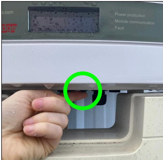
On the A-Style Inverters, the button to activate the screen is in the opening between the top and bottom sections of the inverter.
