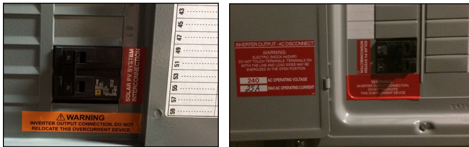
Examples of Interconnection Breakers
