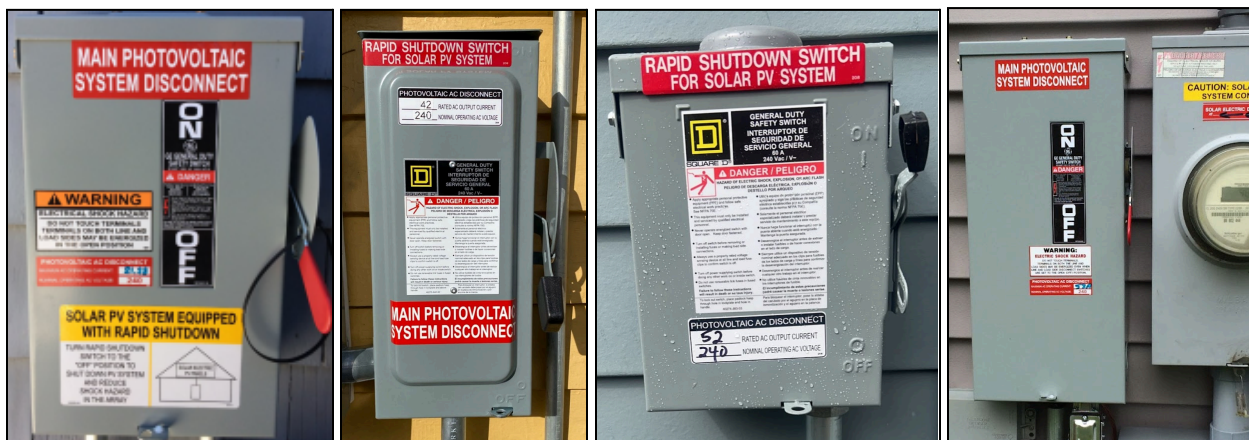
Examples of AC Disconnect Switches
